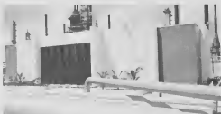
The Refining Operations Center (ROC), from where almost all process units are computer controlled.
